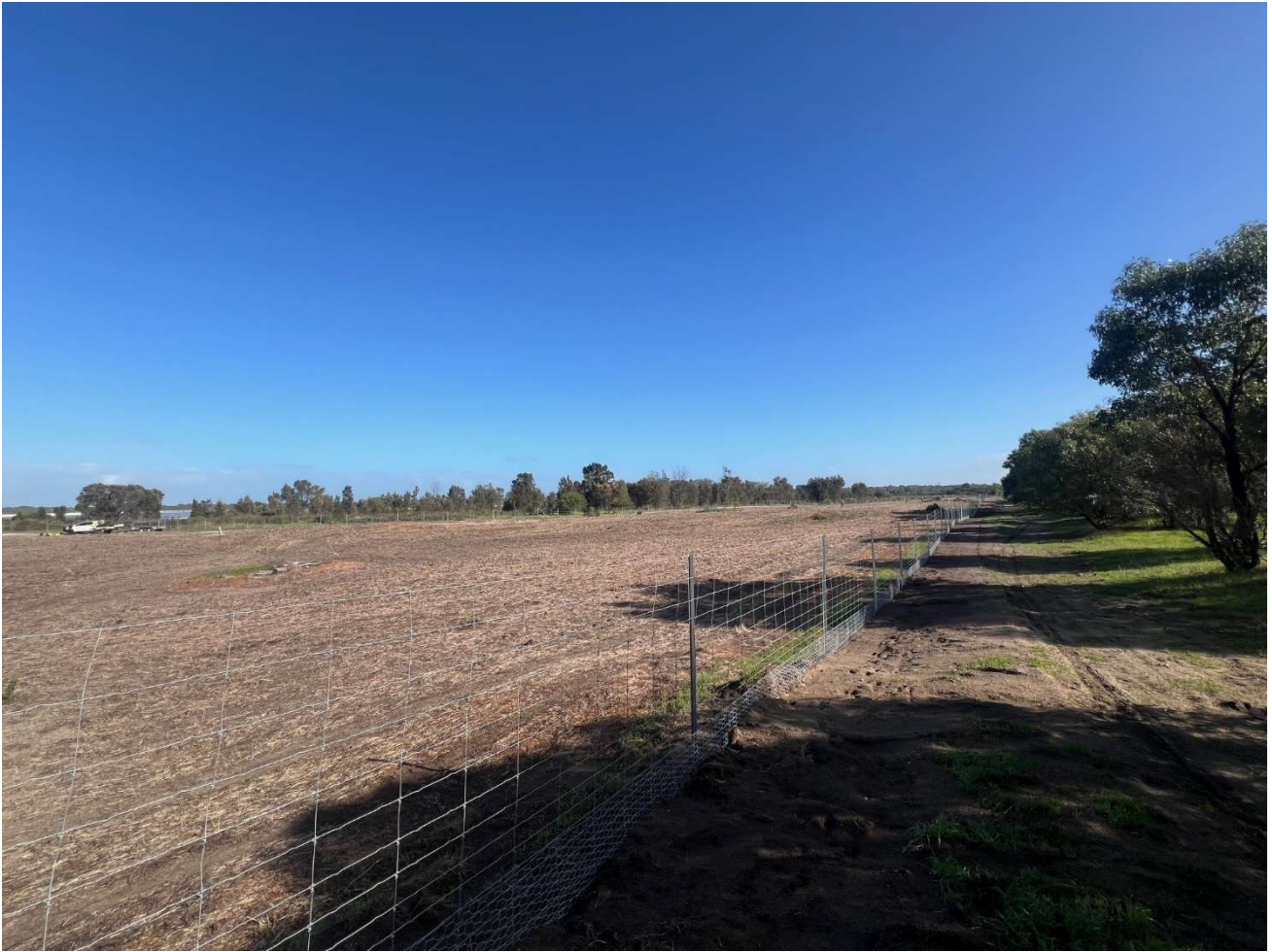
Figure 5: 250710_Rockingham Lakes Revegetation Site_2. Offset Site perimeter fencing.
