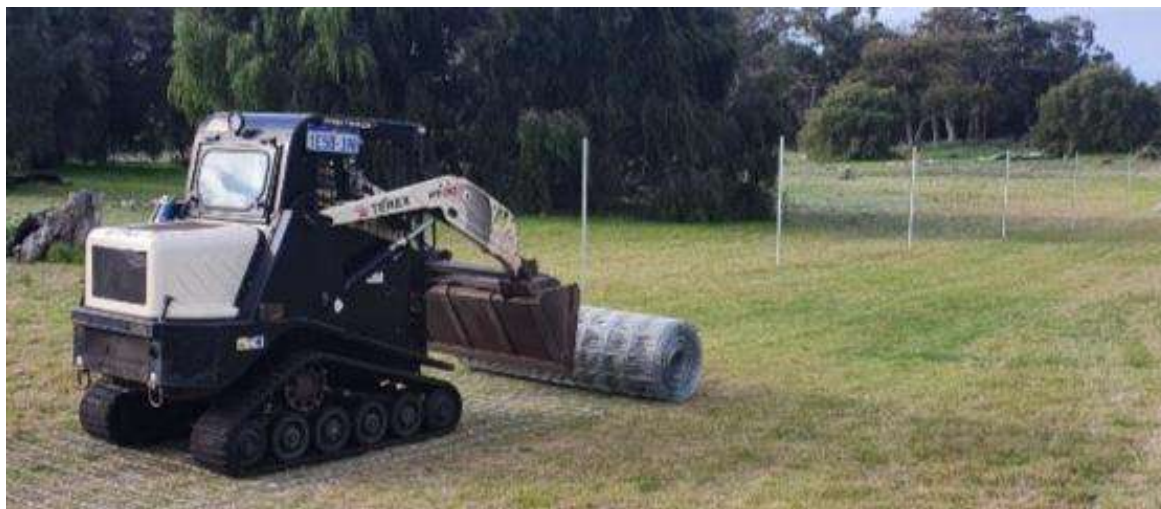
Figure 3: Natural Area's posi-track loader rolling out ringlock mesh along a fence alignment (Shire of Capel).
