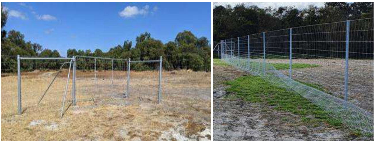
Figure 9: An example of a gate installed ( left ), and installation of rabbit proof netting ( right ) for the Shire of Capel at the Kemerton Offset site.
