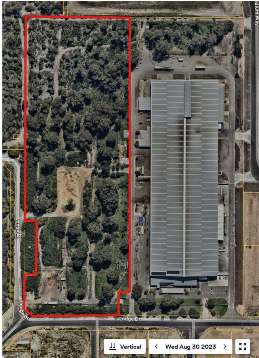
Figure 2:6 Lodge Drive highlighted, with nearmaps website showing the image is from August 30th 2023, before the clearing commenced
